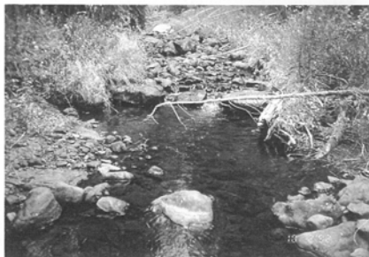
Figure 35—Scour, mid channel, boulder formed (SMB).
