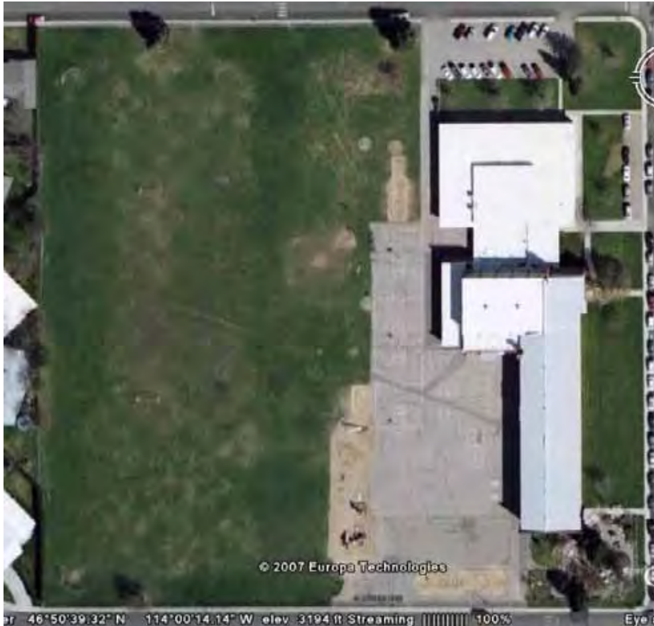
Lewis & Clark Elementary School
