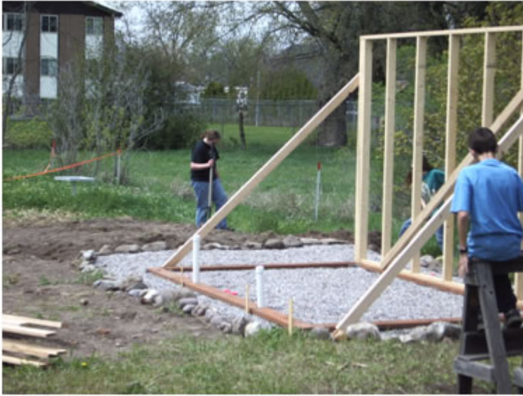
8 th grade greenhouse under construction, Sussex School May 2005
